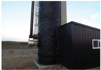
Left: the treater and valve house after the SPF and polyurea applications; Right: SPF and polyurea were applied only on the first 15 feet of the oil treater
