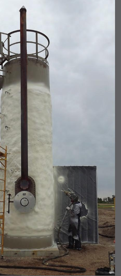
Not only had the treaters' propane consumption remained high, but also the fiberglass became wet over time, which permitted rodents to break through the batt insulation, cancel all R-value and, disdainfully, generate a rodent issue. With a high propane consumption, no air and vapor barrier, inefficient insulation, and a rodent problem to deal with, the oil field owner opted for a solution that would take care of his problems: spray polyurethane foam insulation.
